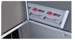
Step 1: Tack/secure the end of the roll with a nail. Unroll the membrane 3–6 feet.
