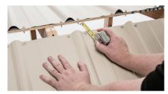
Step 1: Make sure panel is free of dust and debris. If not pre-cut, cut 2" slot at ridge. Measure and mark where the ridge cap will sit on the panel.
