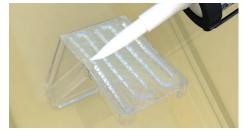
Step 1: After cleaning the metal roof surface, apply a sealant to the back surface of the Yeti Guard.
