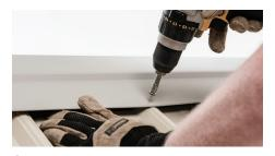
**Step 3:** Apply ridge cap, compressing material between the ridge cap and major rib. Fasten at the major rib using a screw gun set to at least 2700 rpm.
