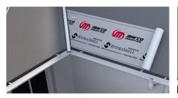
Step 1: Tack/secure the end of the roll with a nail. Unroll the membrane 3–6 feet.
