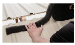
**Step 2:** Start from the end of the ridge, rolling out Flex-O-Vent along the length of the ridge (both sides), making sure the vent sits "up-slope" from the edge of the ridge cap.
